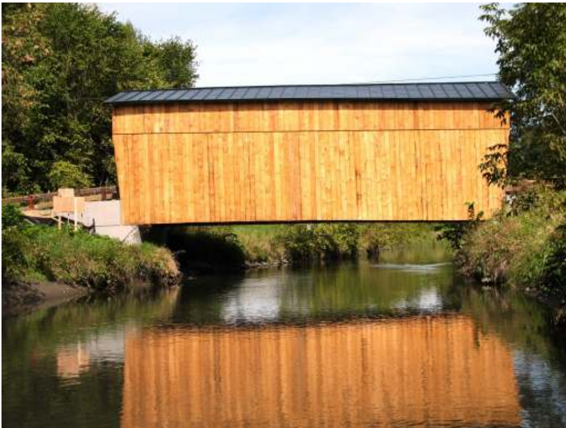
*Randolph TH 60, bridge 40 (Kingsbury Covered Bridge)
