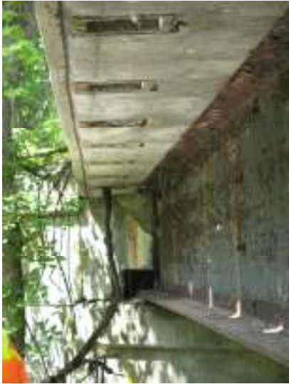
*paint deterioration
