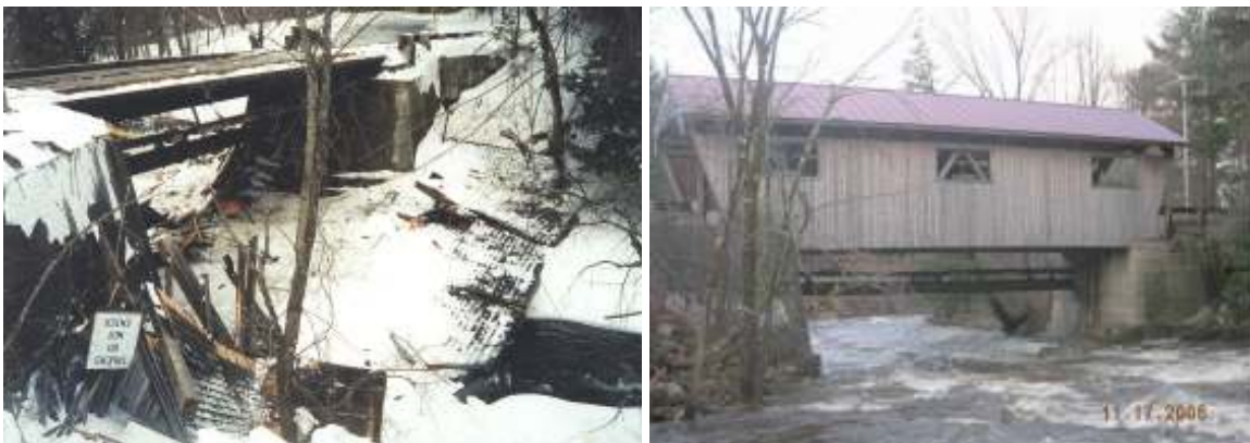
*Johnson TH 3, bridge 4 (Power House Covered Bridge) – before and after
