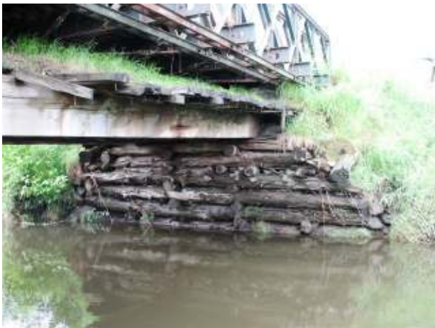
*Craftsbury TH 59, bridge 2 – before
