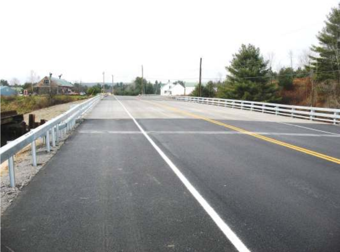
*East Montpelier US 2, bridge 74 (Carpet Barn Bridge)
