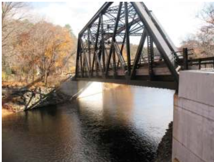
*Springfield TH 66, bridge 81
