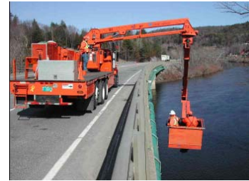
Bridge inspection equipment
