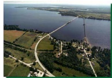
Missisquoi Bay Bridge Rt. VT 78 over Lake Champlain
