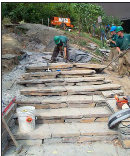
VYCC crews have assisted with the construction of the Statehouse Path in Montpelier
